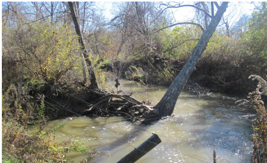
Photo 2: Exposed clay in eroding bank segment and high turbidity conditions in Spring Brook near the Tompkins County line.
