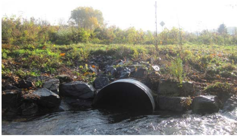
Photo 10: Direct conveyance of runoff into Taughannock Creek from nearby roads and farm fields.
