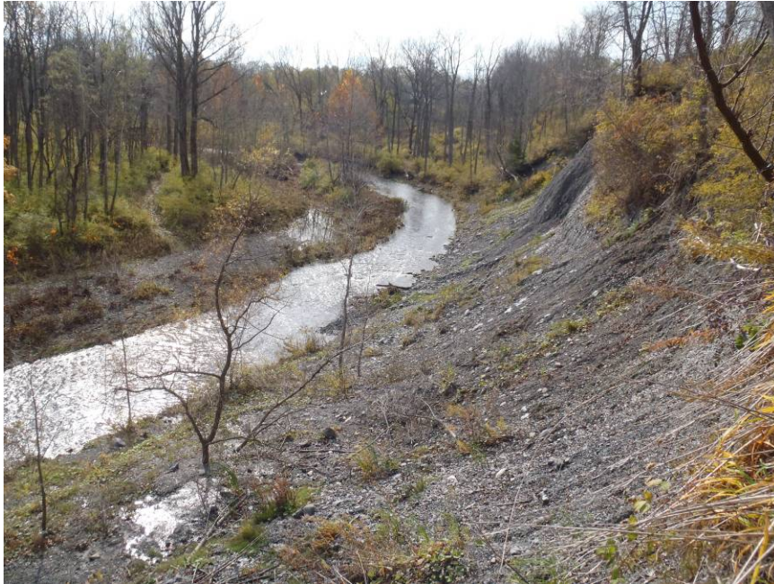
Photo 5: Facing upstream at the downstream end of the South Street Extension bank failure site.
