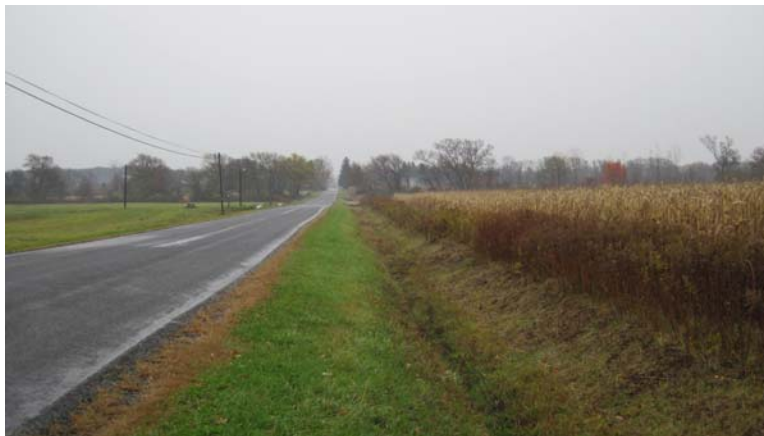
Photo 11: Vegetated agricultural ditch conveying runoff to a nearby stream.
