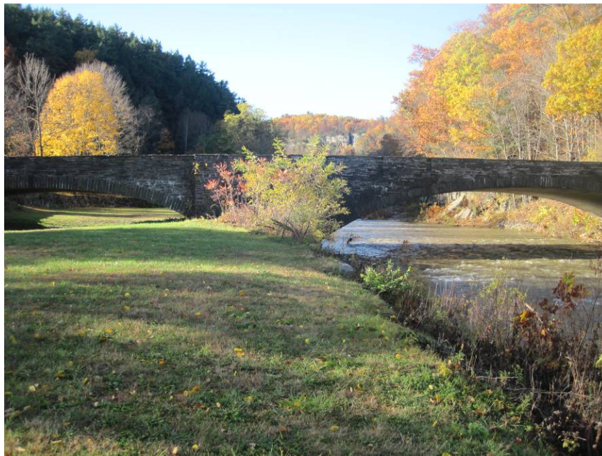
Photo 9: Route 89 Bridge showing turbidity in main channel (facing upstream).
