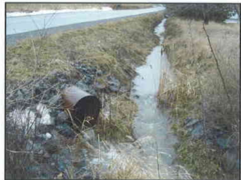
Lansingville Road – Culvert 5. Start of hedgerow stream.
