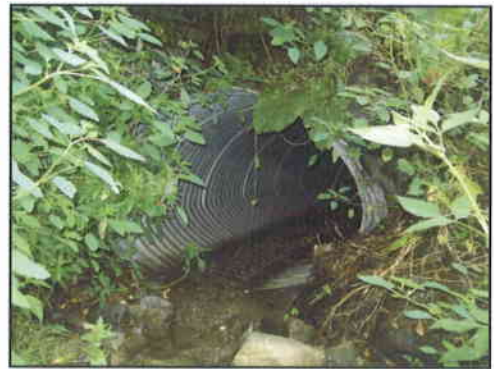
Ludlowville Road Culvert 12
