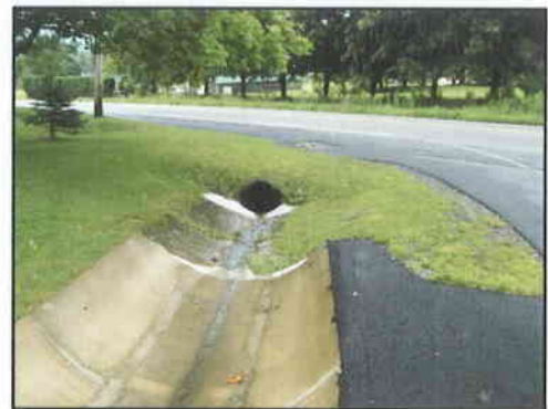
Transition from open to closed drainage at Lansingville/Ridge Road intersection.
