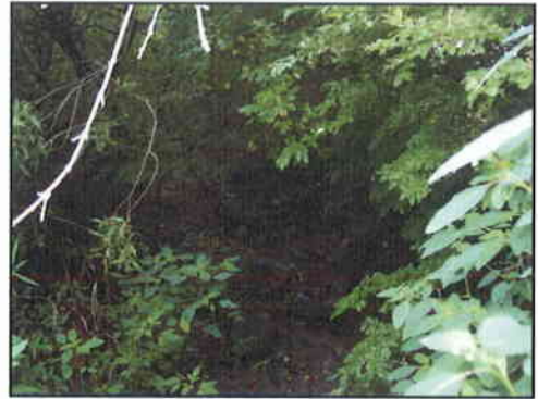
Open channel drainage upgradient of Ludlowville Road Culvert 12.
