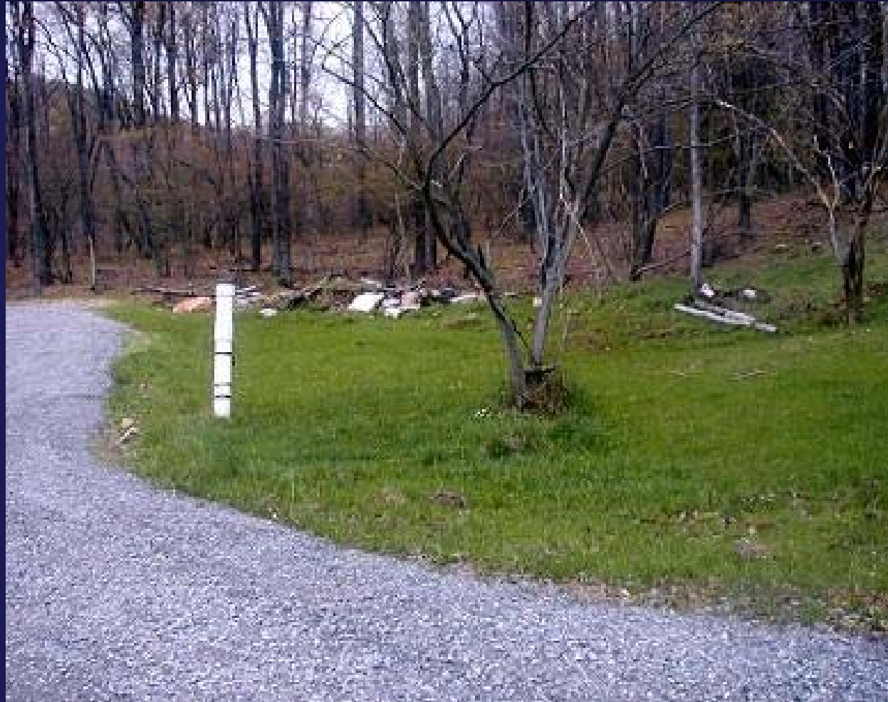
Bioretention / Infiltration Area
