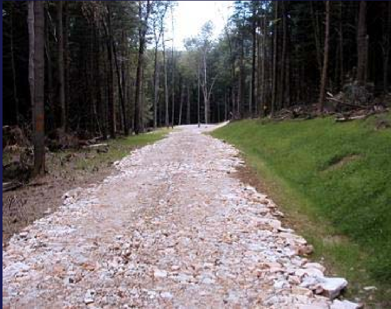
Stabilized road surface
