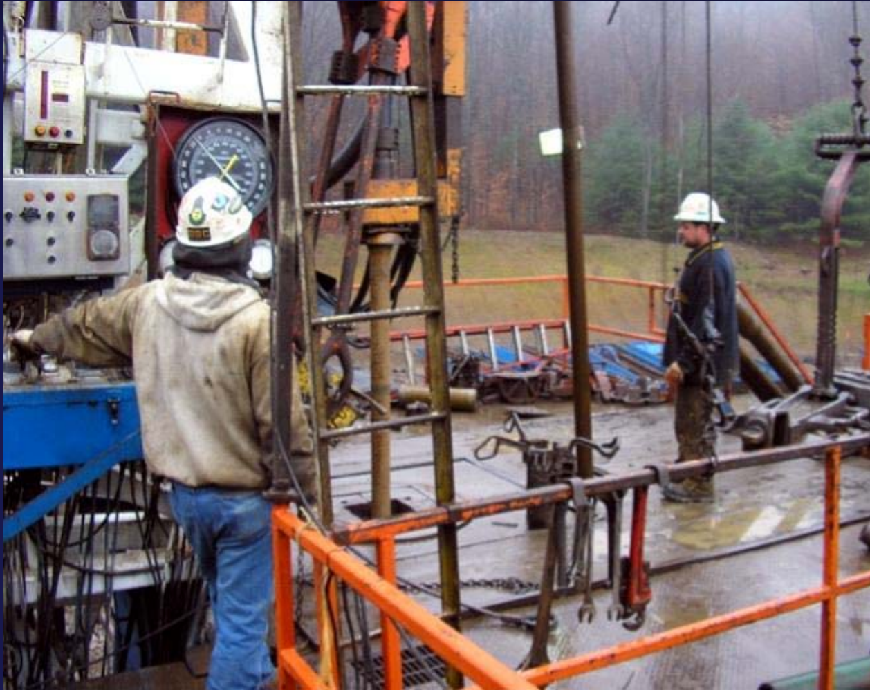
Drilling the Well
