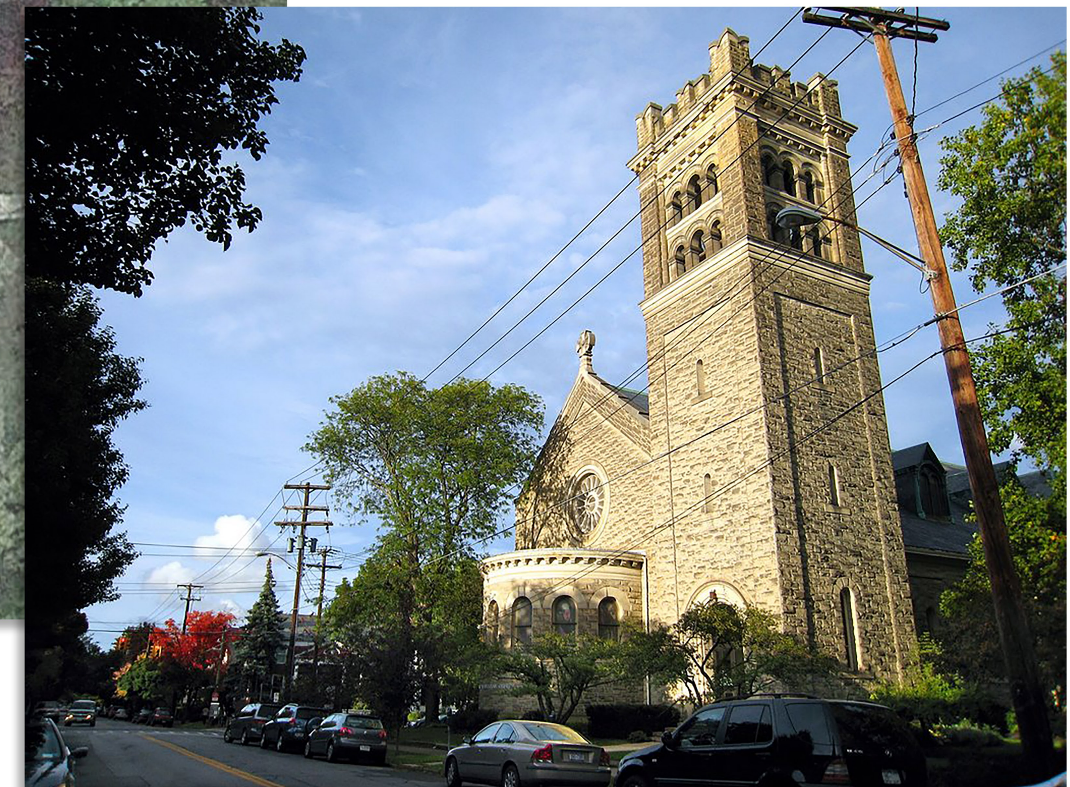
FIRST PRESBYTERIAN CHURCH - VIEW FACING NORTH ON N. CAYUGA STREET
